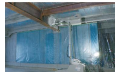
Fireproof coating sprayer robot (smart construction technologies)
