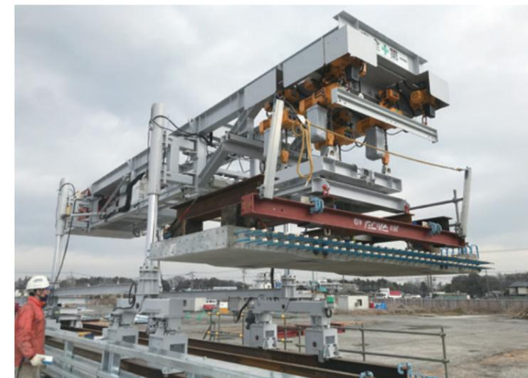
SDR System demonstration test. Machine to install precast slab
