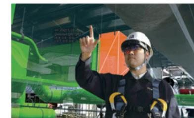
Checking the construction alignment by overlaying the actual product and BIM (BIM utilization)
